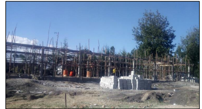
The new building under construction
